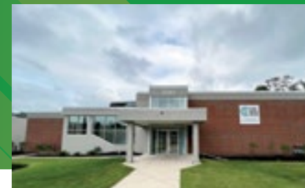
The lab in Harrisburg is one of the recent additions to the Clean Energy Center's training sites, equipping individuals with the skills to weatherize homes and buildings in their communities.
