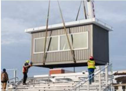
Press Box Installed at Wildcat Athletic Field
