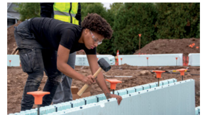
Shanya M. Allen, a building construction technology student, taps a second course of insulated concrete forms to interlock with the first.
