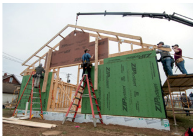
Top of page: Residential construction technology & management students Charli Spradlin (left) and Cassandra Guiffre plumb a corner guide for insulated concrete forms. Below: Students set trusses (left) and sheathe the roof.
