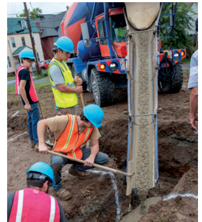
Students in a Concrete Construction class pour the home's footer.
