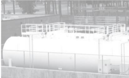
**UL-142 Double Wall Storage Tanks for Wayne Memorial Boiler and Back Up Generator**
